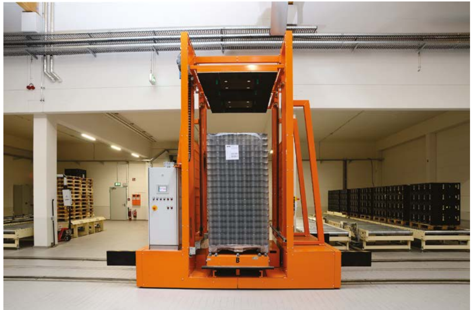
Fully automated pallet handling without forklift traffic.
